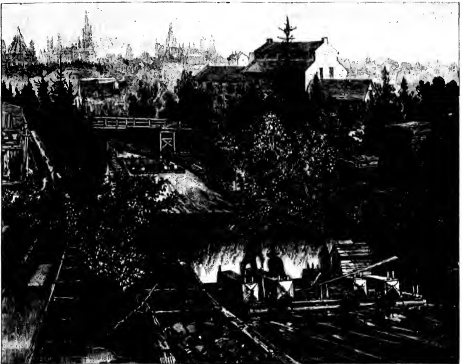
CRIB OF TIMBER RUNNING THE SLIDE.
